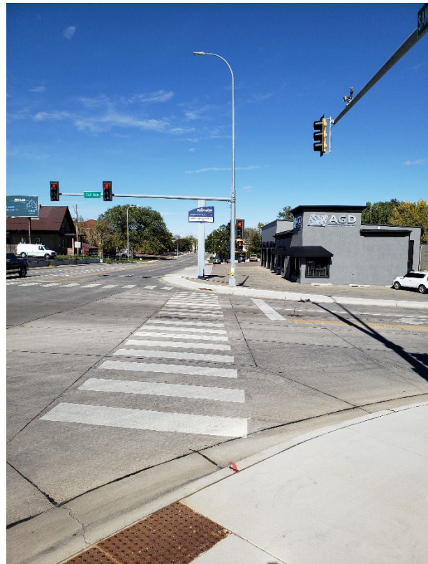
Continental Crosswalk, ADA Accessible Curb Ramps, and Detectable Warning Surfaces at Sanborn Boulevard & 1 st Avenue Intersection
